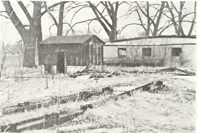
The post factory west of Lock 17 where concrete fence posts and telephone poles were manufactured, c. 1970. All that remains today are the factory's foundations. (Photograph courtesy of Hennepin Canal Parkway.)
